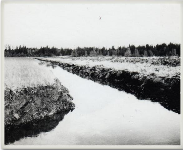
**Figure 4.** Construction of the canal that drained Lake Västervikssjön. Photos from around 1956, by Abel Åberg.
