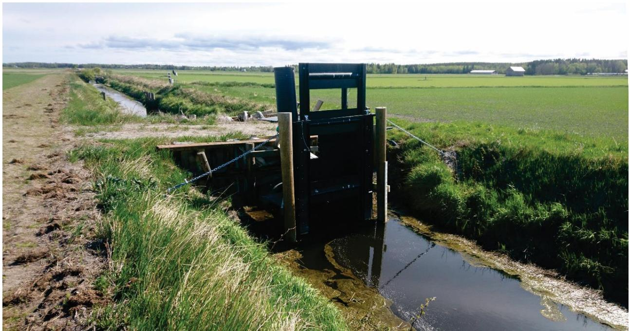
**Figure 4.** The SBDam, constructed to ensure access to irrigation water during the summer. Photo: Peter Österholm.
